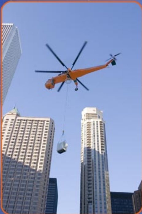
The Aircrane can place over 100 HVAC units per day.
